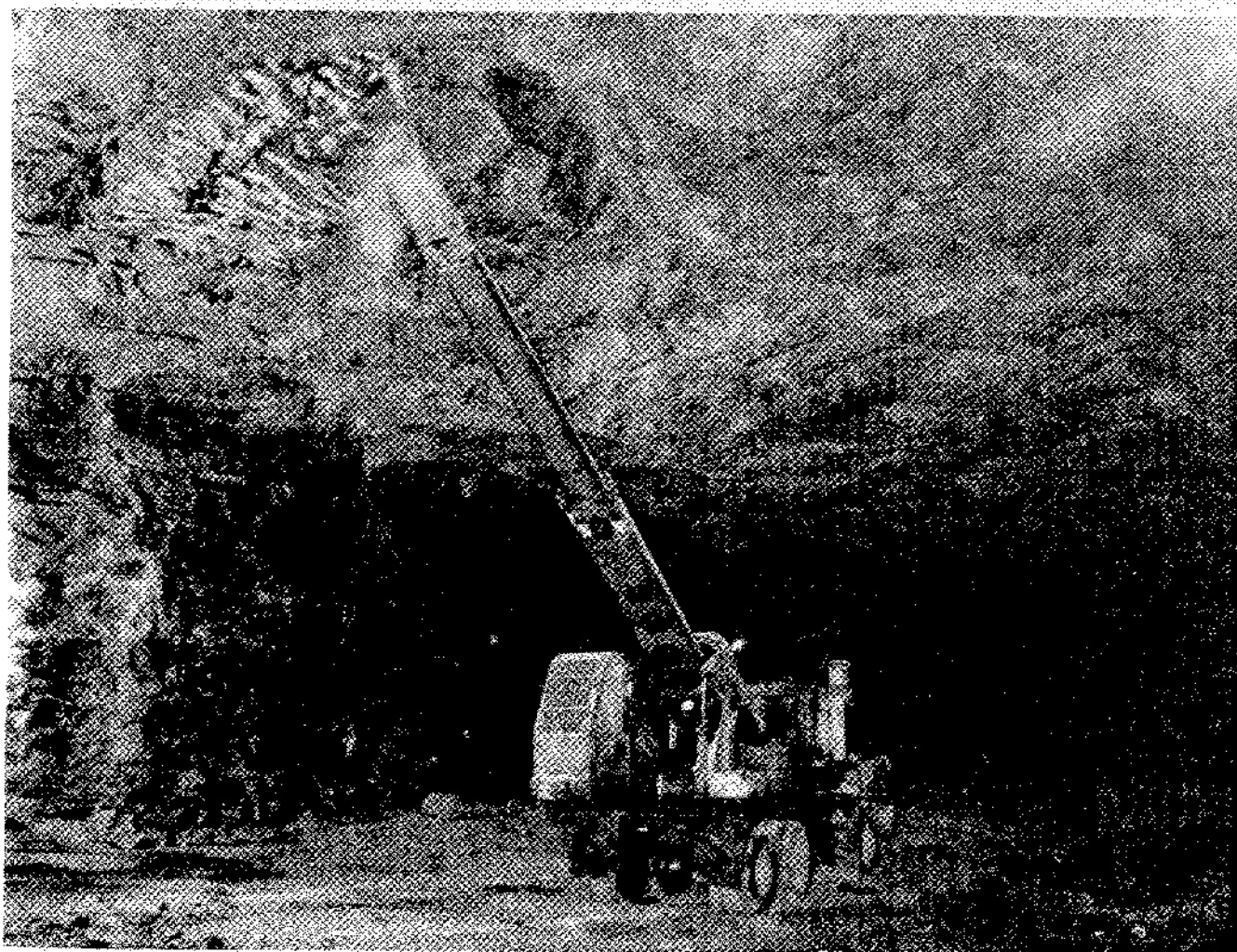
Figure 2: Scaling with Gradall Machine.
